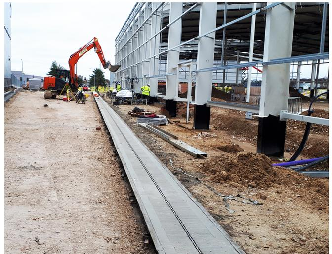
Once installed in the ground if it is necessary for site equipment to traverse the trench, a protective bridge should be formed to protect the Swarm Aqua® channel from unnecessary damage. It is important that Swarm Aqua® is never trafficked prior to the final stage of it's installation, as the strength of the drainage channel is dependent on it's concrete surround and any unnecessary loading will cause deformation and may affect the quality or length of the channel's lifespan
